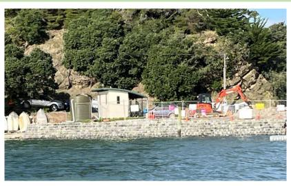
Work is well advanced on rebuilding and stabilising the seawall next to the carpark at Scott Point. The northern side of the wall is expected to be completed in the next few weeks and clearing material and breaking into the bedrock for the foundations on the southern side will proceed as tides permit. Once work on the seawall is complete, the car park will be redesigned and re-surfaced with the establishment of boat trailer parks.
