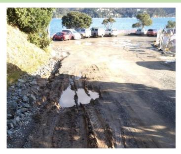
The heavy vehicle movements associated with the seawall upgrade have further highlighted the precarious state of the gravel section of Ridge Road, which has suffered further damage from weather events this year. MERRA has been in ongoing dialogue with Auckland Council and Auckland Transport to ensure that the necessary remedial work is undertaken to stabilise the slips and prevent further sediment entering the harbour.
